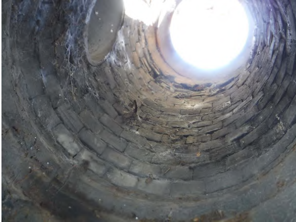
Figure 1 – STA. 10+00 24-inch Manhole at Grant Street.
