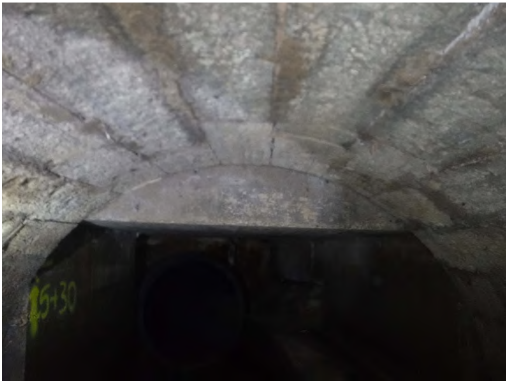
Figure 18 - STA. 15+30 railroad arch bridge structure.
