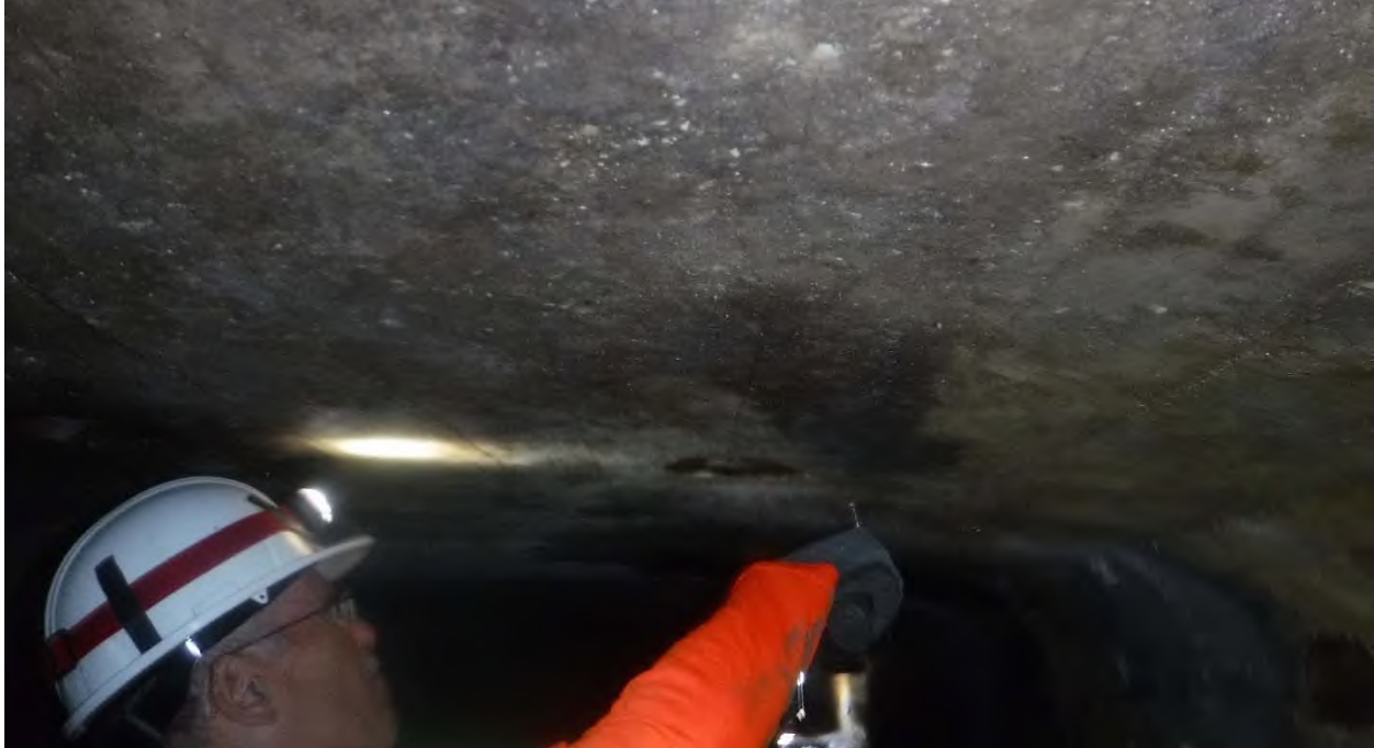
Figure 6 – Sounding concrete for voids with roofing hammer.
