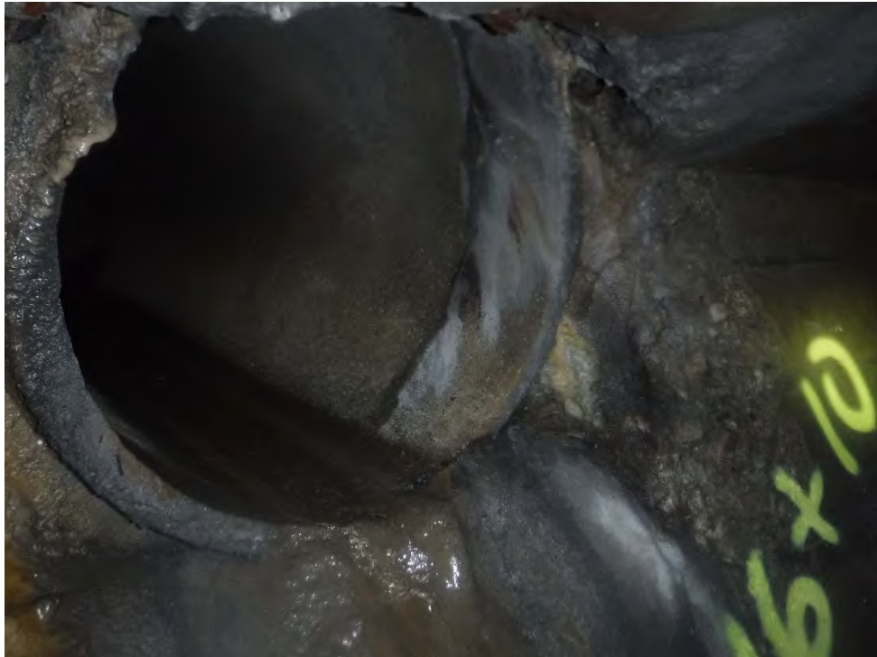
Figure 26 - STA. 16+10, 18" Concrete connection.
