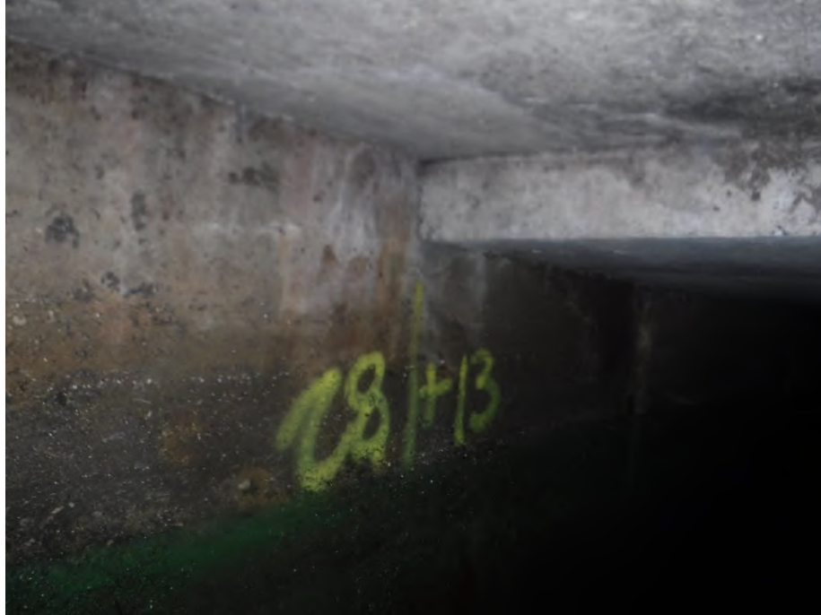
Figure 95 - STA. 28+13 construction joint.
