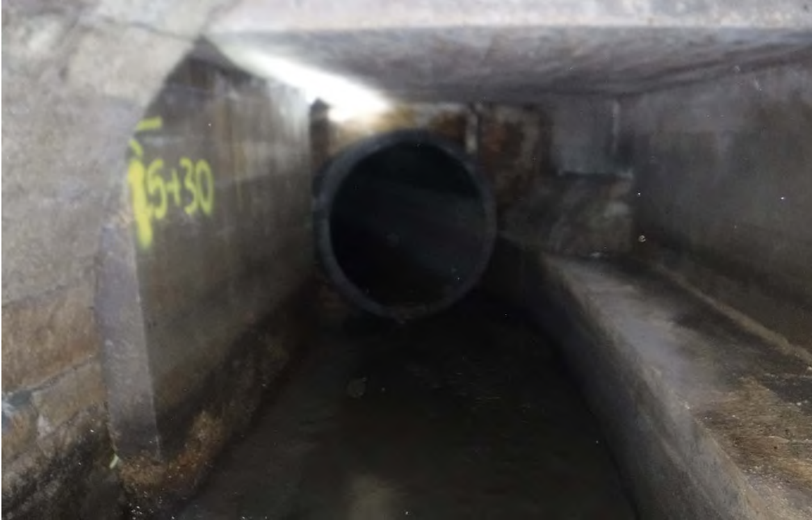
Figure 4 – 48-inch diameter HDPE storm sewer at Station 11+32 (facing north)
