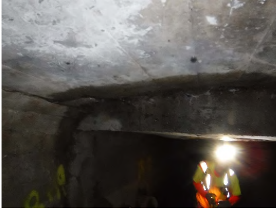
Figure 44 - STA. 18+19 construction joint.
