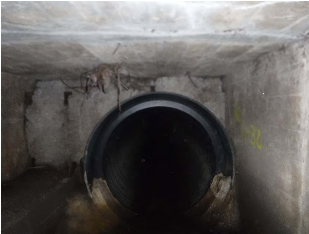
Figure 14 - STA. 11+32, 48-inch diameter storm sewer lining.
