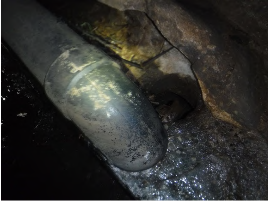
Figure 79 - STA. 21+26 open sanitary sewer connection.
