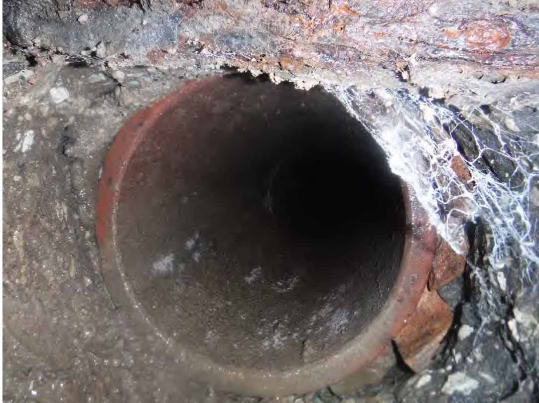
Figure 65 - STA. 20+28 8" clay connection.
