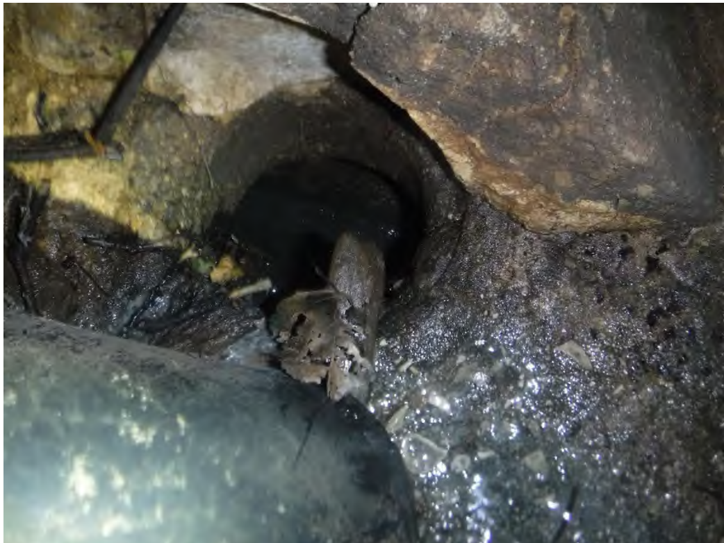
Figure 78 - STA. 21+26 open sanitary sewer connection.
