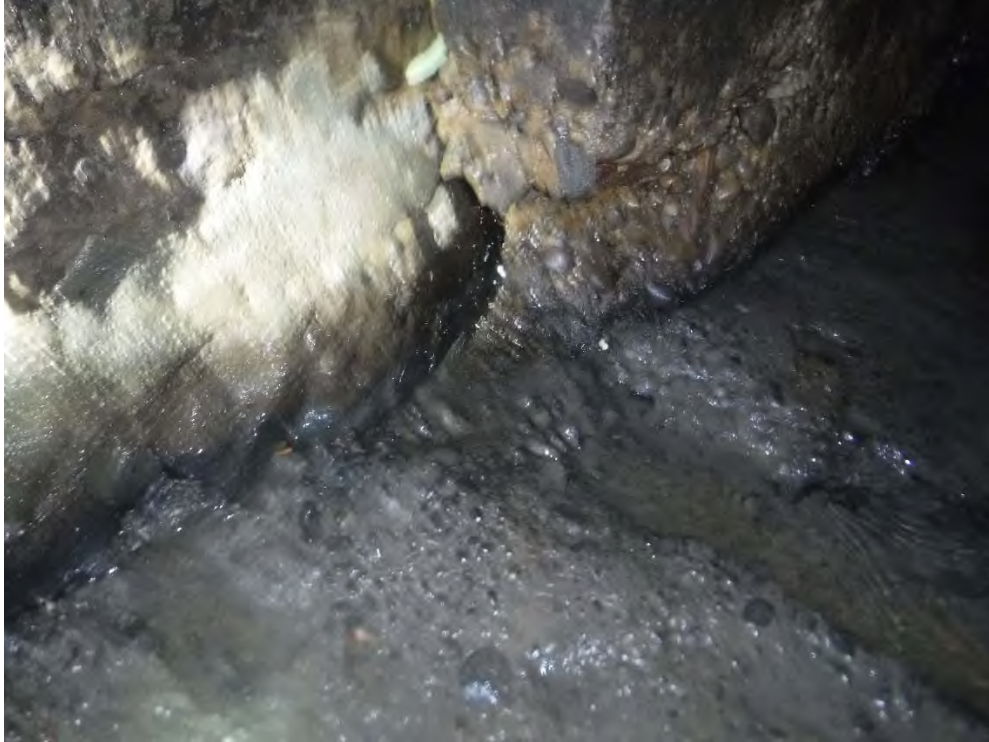
Figure 19 - STA. 15+30 infiltration.
