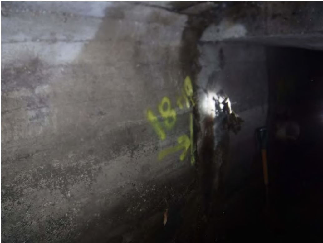
Figure 45 - STA. 18+19 construction joint.
