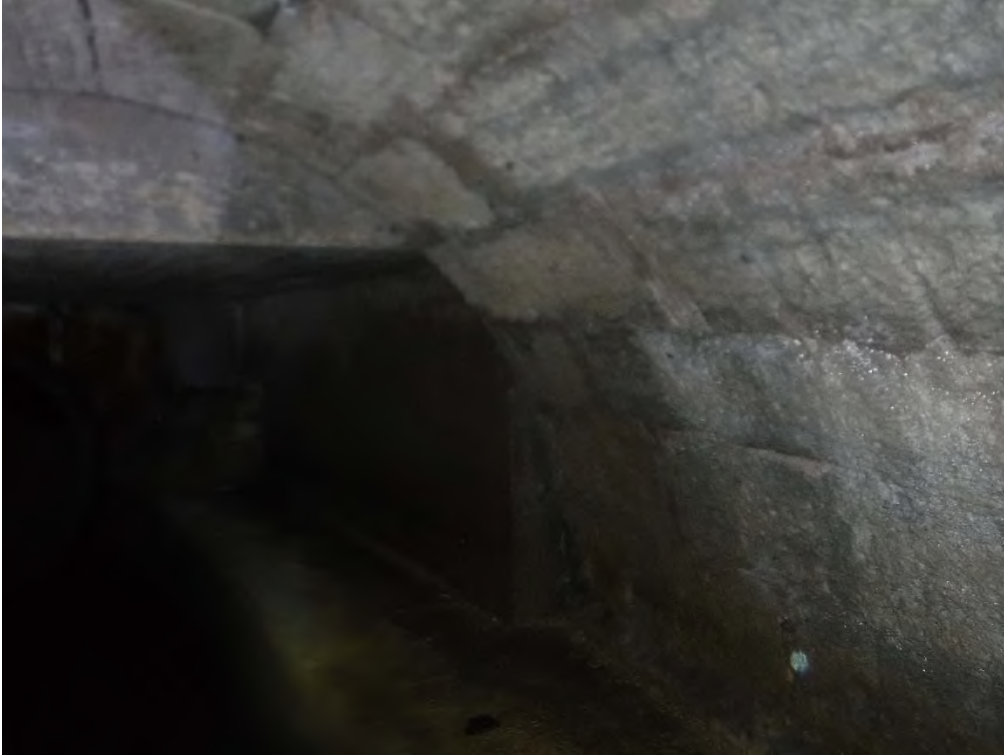
Figure 17 - STA. 15+30 railroad arch bridge structure.
