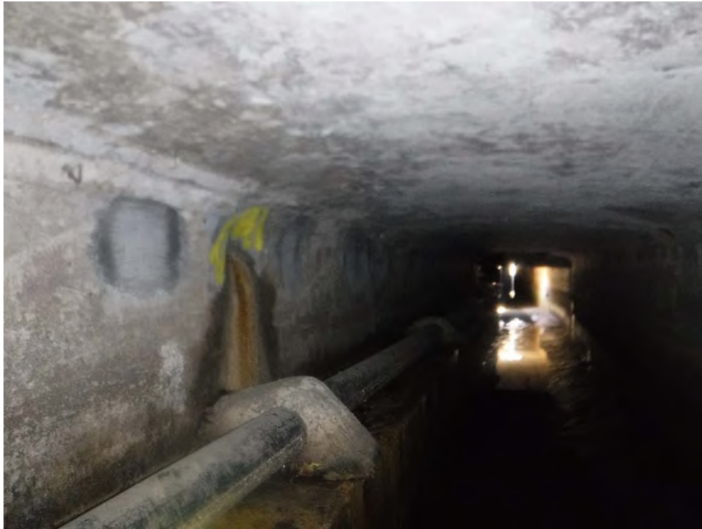
Figure 7 - Field investigations of the culverts on July 13, 2022.
