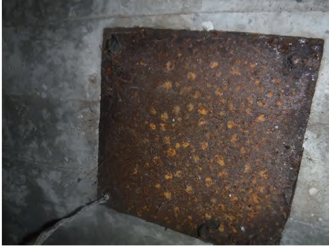
Figure 57 - STA. 19+36 steel plate repair in ceiling.
