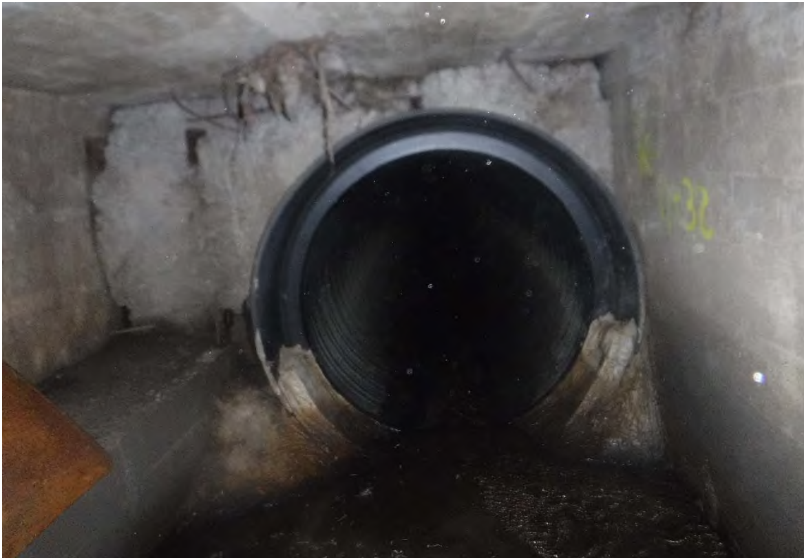
Figure 4 – 48-inch diameter HDPE storm sewer at Station 11+32 (facing north)
