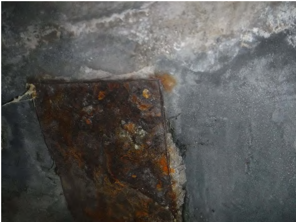
Figure 47 - STA. 18+63 Ceiling patch.
