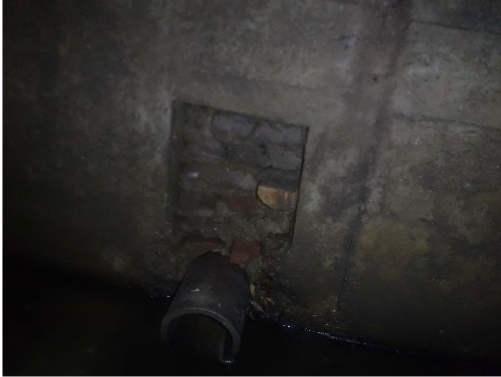
Figure 11 - STA.10+90 6" DI. Recommended grout connection.
