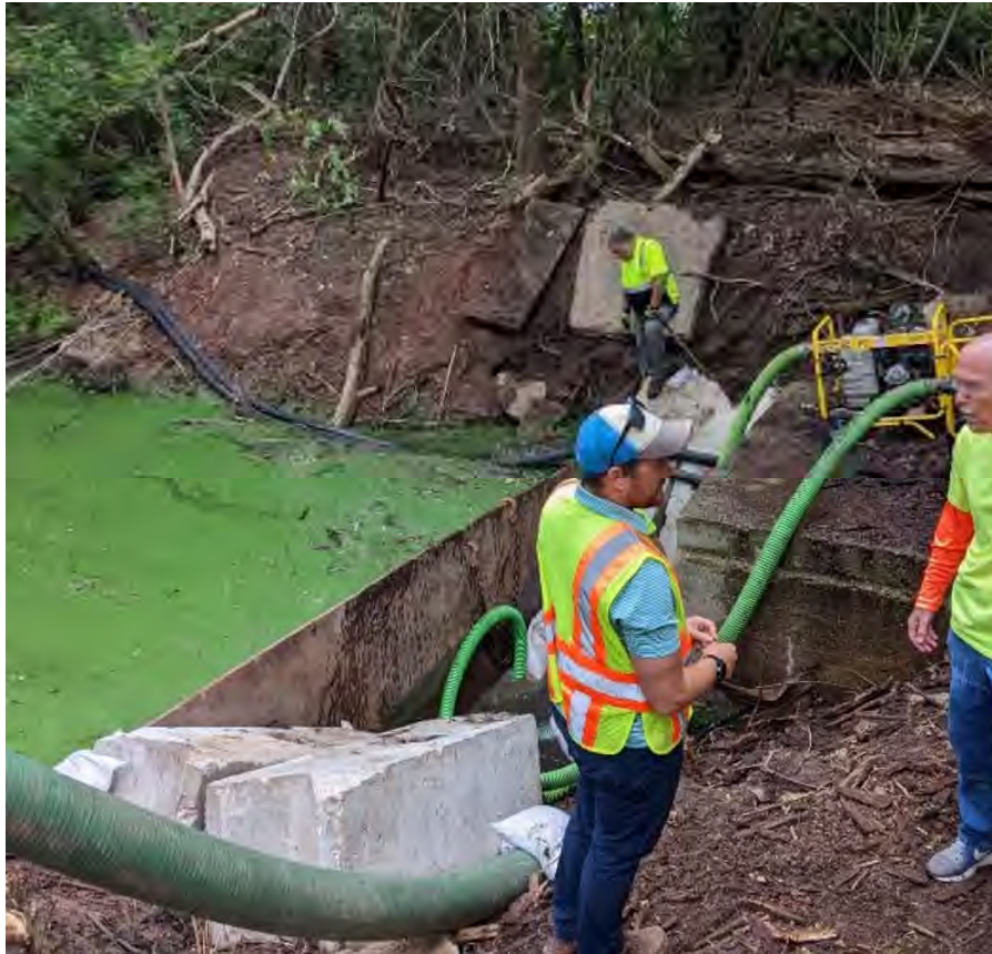
Figure 5 – Dewatering operations at the outfall at Fox River on July 13, 2022.
