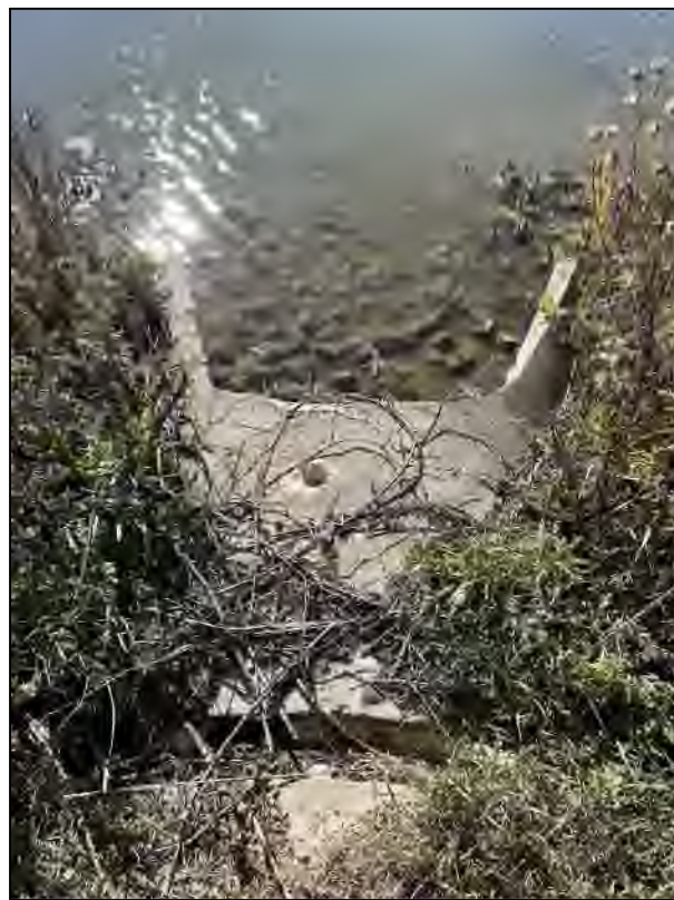
1. REPAIR EXISTING ENDWALL ON ROCKLAND POND OUTFALL FOLLOWING JOINT TIES DETAIL ON SHEET C507
