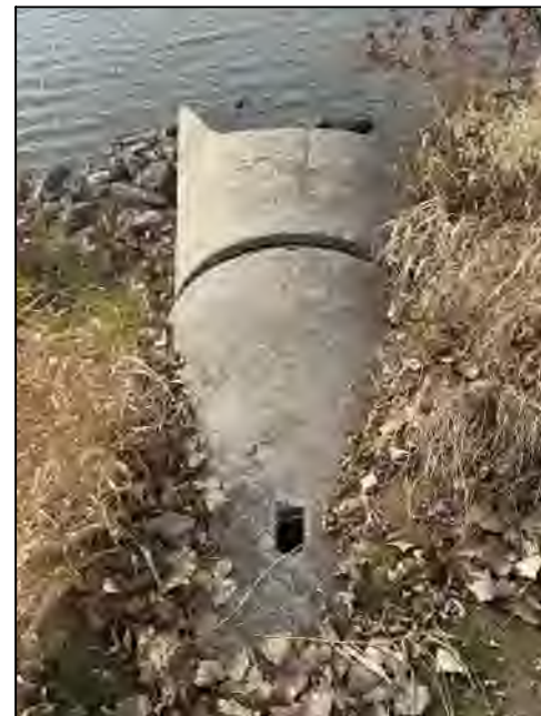
2. REPAIR EXISTING ENDWALL ON SADDLEBROOK LANE POND OUTFALL FOLLOWING JOINT TIES DETAIL ON SHEET C507
