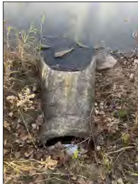
2. REPAIR EXISTING ENDWALL ON SADDLEBROOK LANE POND OUTFALL FOLLOWING JOINT TIES DETAIL ON SHEET C507
