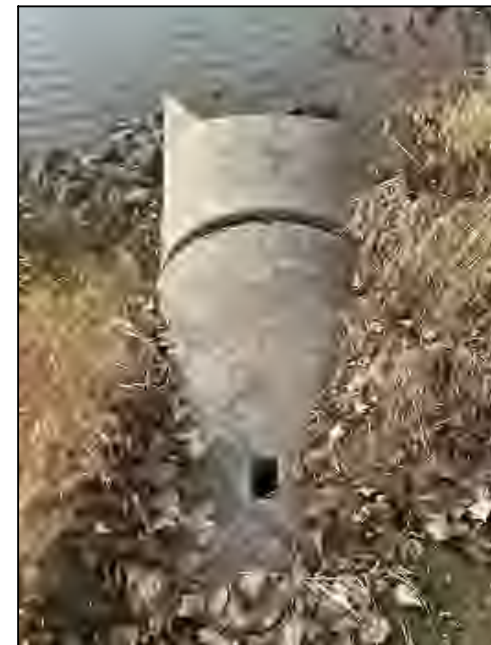
2. REPAIR EXISTING ENDWALL ON SADDLEBROOK LANE POND OUTFALL FOLLOWING JOINT TIES DETAIL ON SHEET C507
