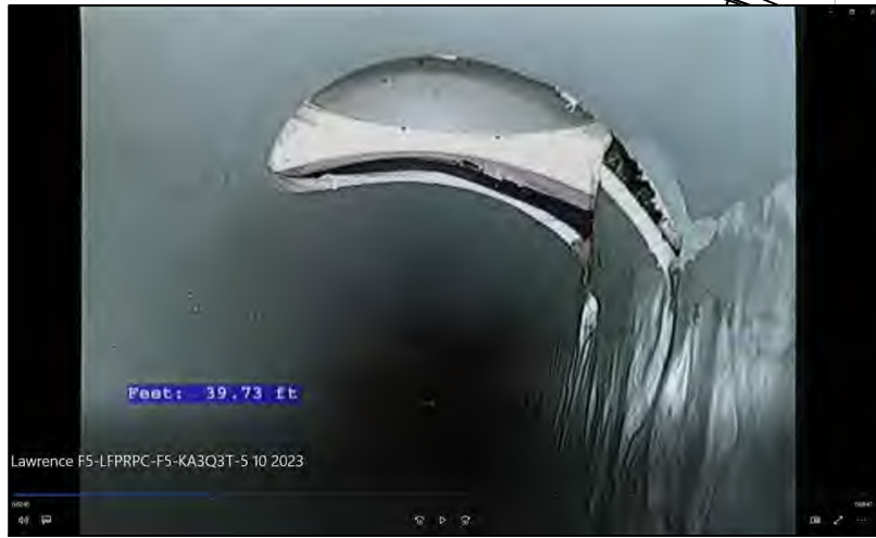
OVER CUT STORM LATERAL REQUIRING CONCRETE COLLAR
